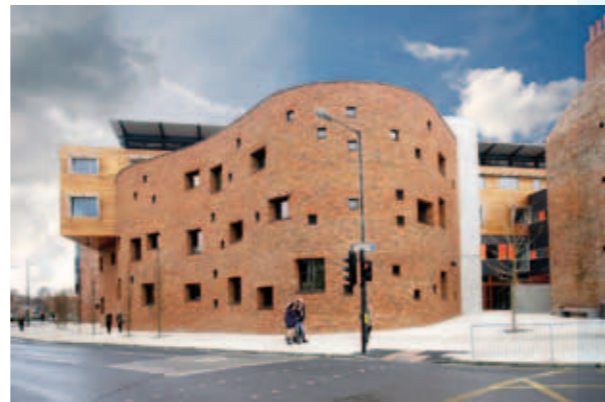
Award winning building Students learn in a simulated environment (top image). ALPS capital funding supported the development of the iconic and award winning De Grey Court building (above and right).
